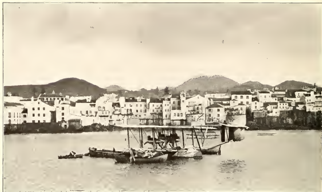
THE NC-3 AT PONTA DELGADA. NOTICE THE NAVAL CUTTERS PLACED UNDER HER WINGS TO PREVENT CAPSIZING
